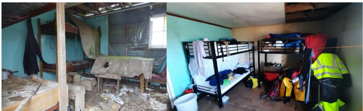
Figure 2: The existing shanty was derelict with a missing door, collapsed ceilings and an open roof on the windward side. Turkey vultures were living inside. The structure has been repaired, re-roofed and now provides dry and draught-free sleeping for 4 people.
